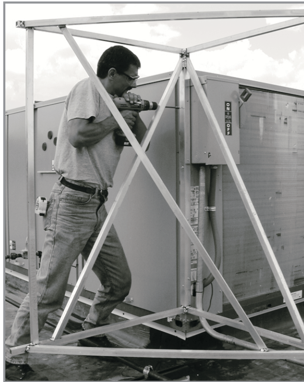
CORNER TRUSS INSTALLATION
