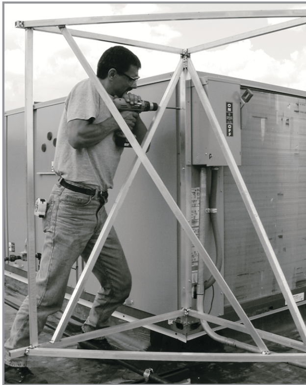
CORNER TRUSS INSTALLATION
