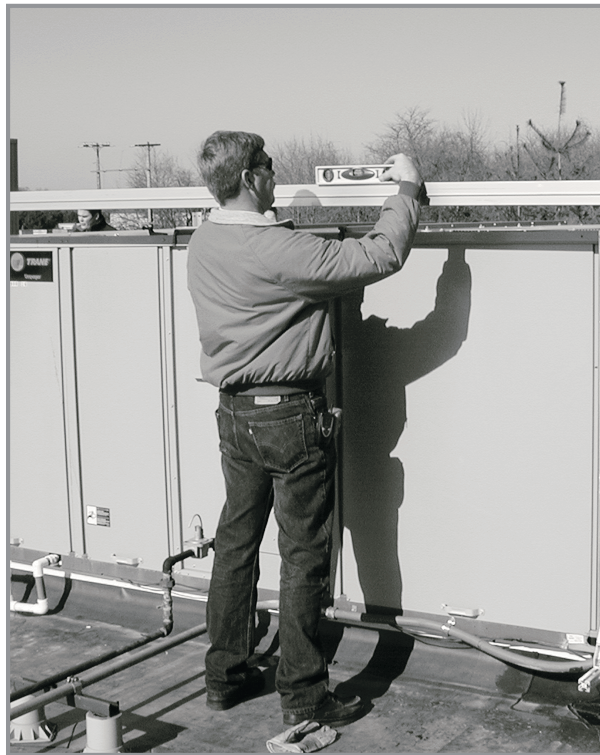
LEVELING THE COMPONENTS
