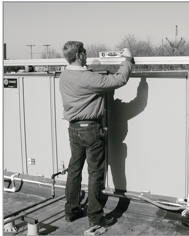
LEVELING THE COMPONENTS
